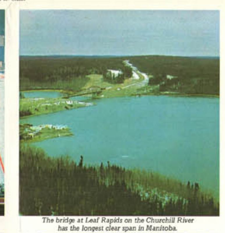
The bridge at Leaf Rapids on the Churchill River has the longest clear span in Manitoba.
