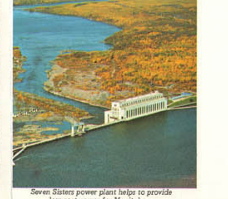
Seven Sisters power plant helps to provide low-cost power for Manitoba.
