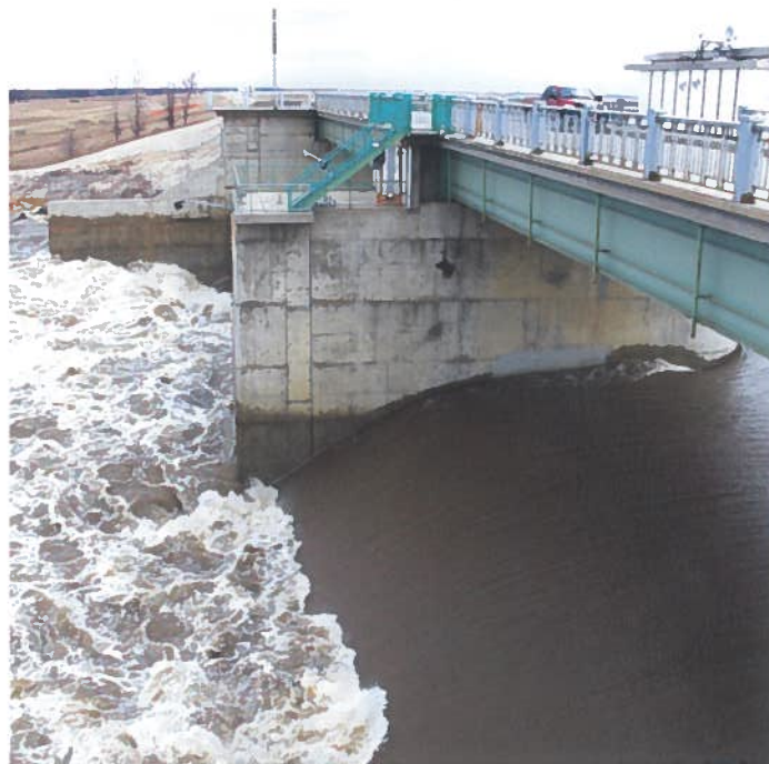
Floodway inlet control structure south of Winnipeg
