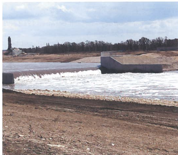
Floodway outlet structure north of Winnipeg
