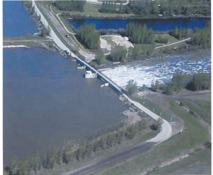
Portage Diversion structure
