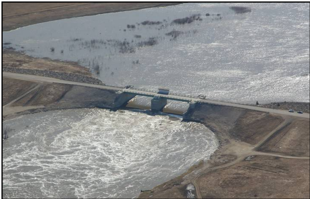
PHOTO 2-3 – INLET CONTROL STRUCTURE DURING SPRING 2004 OPERATION ( Q=1470 \text{ m}^3/\text{S} )
