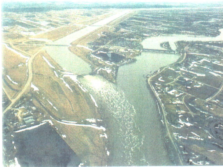
Photo 6: Looking upstream along Floodway Channel (left) and Red River Channel (right). Floodway Outlet Structure in left centre.
